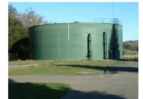
Chlorine Contact Tank (capacity 750,000 gal)
